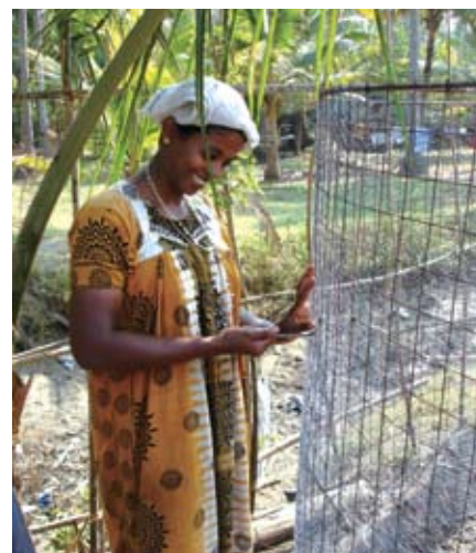
Beneficiary assisting with construction of RWH tank, India
