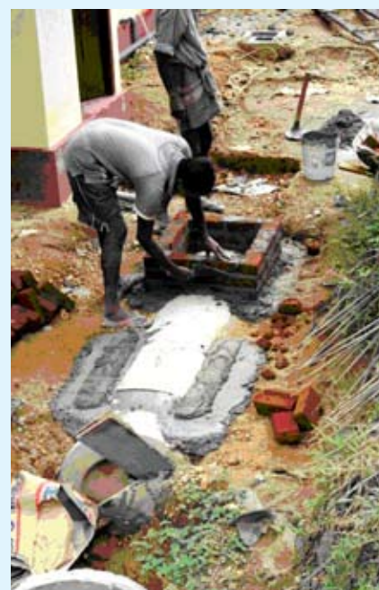
Construction of septic tank, control chamber
