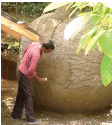
Rainwater harvesting tank under construction in Ransagoda, Matara District, Sri Lanka
