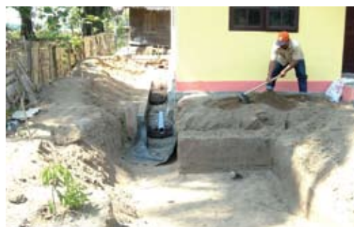
Construction of a wetland and leach field where the pre-treated effluents from the Biofil tank are further filtered and finally released into the ground, Indonesia
