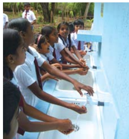
Child friendly school WASH facilities in Ampara District constructed in collaboration with UNICEF, Sri Lanka
