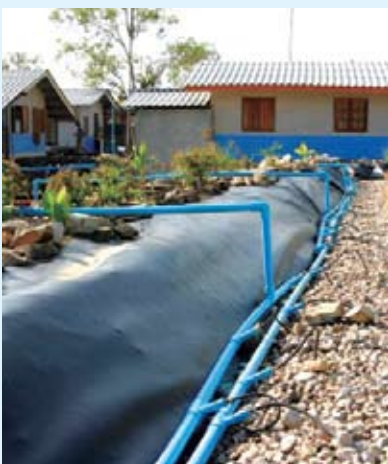
Wastewater pumped into sub-terra reed bed
