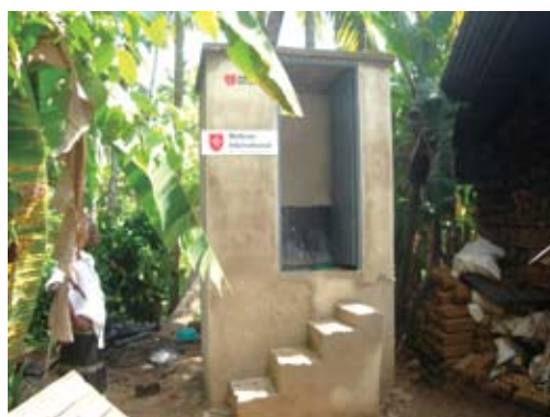
Compost latrine in Habaraduwa, Sri Lanka
