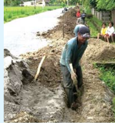
Trench digging in progress for pipe laying
