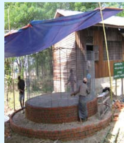
School RWH tank under construction
