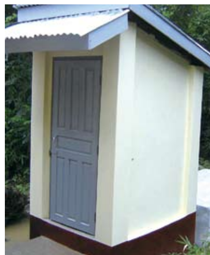
Latrine construction, Myanmar
