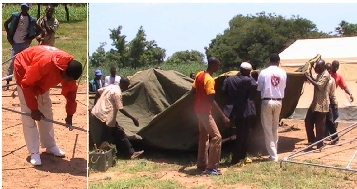
Order of Malta France workers erect temporary tent constructions to benefit victims of the flooding in Kamdomba, Burkina Faso.
