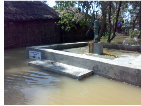
Village well raised above flood water levels
